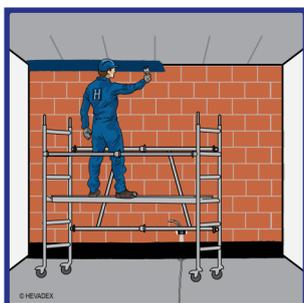
**Wall/ceiling connections** are easily and quickly sealed with Blowerproof brush or spray even on different types of material such as brick, concrete or steel. Different materials react differently to changes in humidity and temperature, which can lead to small cracks in plaster or other finishes leading to air leaks. Applied in two coats second coat must only be applied when the first coat has turned completely black.
